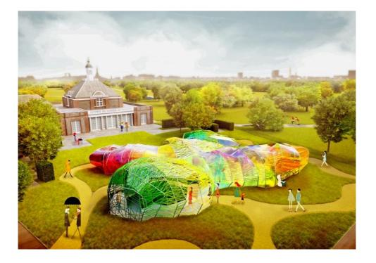
Serpentine reveals today designs for the 15th annual Pavilion. The render by Madrid-based architects SelgasCano shows an amorphous, double-skinned, polygonal structure consisting of panels of a translucent, multi-coloured fabric membrane (ETFE) woven through and wrapped in webbing.
